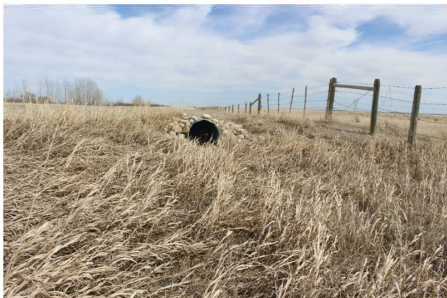
Roadside ditch with culvert near Frank Lake
